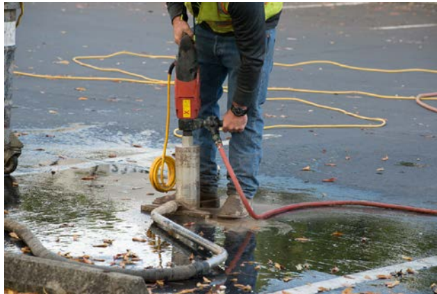
Figure 6: Drill the hole for the PlacePod
